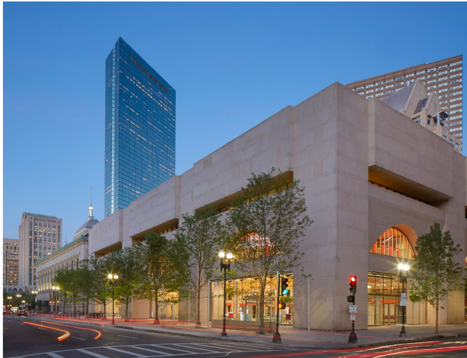
Boston Public Library - Central Branch Johnson Building Improvements Boston, MA
