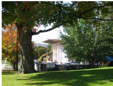
'62 Center for Theatre and Dance at Williams College (under construction)
