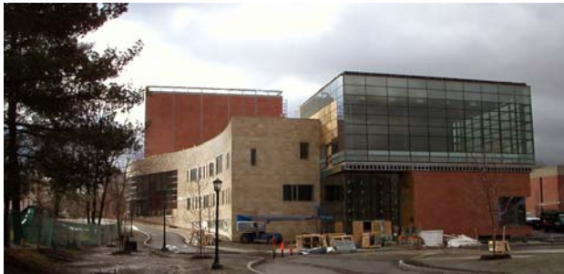
'62 Center for Theatre and Dance at Williams College (under construction)
