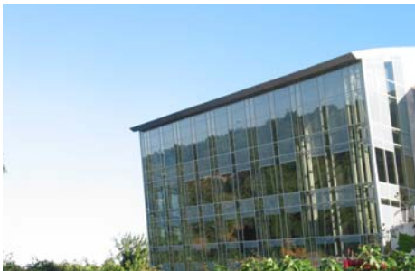
North Lobby at the Music Center at Strathmore
