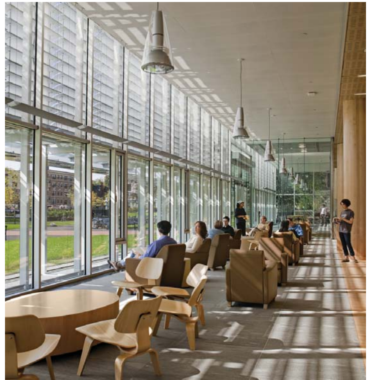
Double-skin wall ensures thermal comfort for patrons along column-free perimeter
