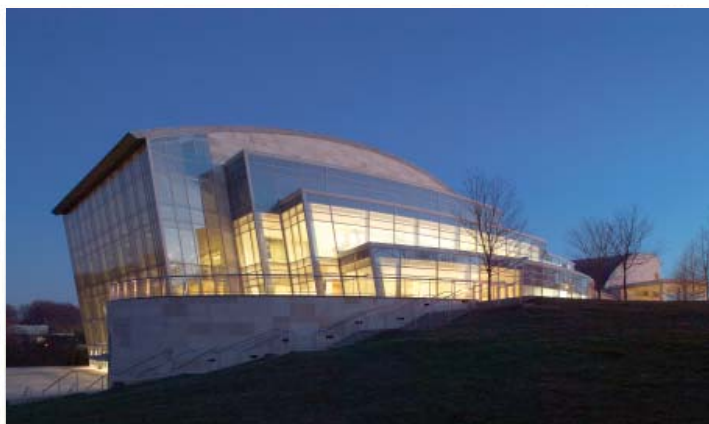
The west elevation of the concert hall features three bulging, stepped facades made mostly of glass.
